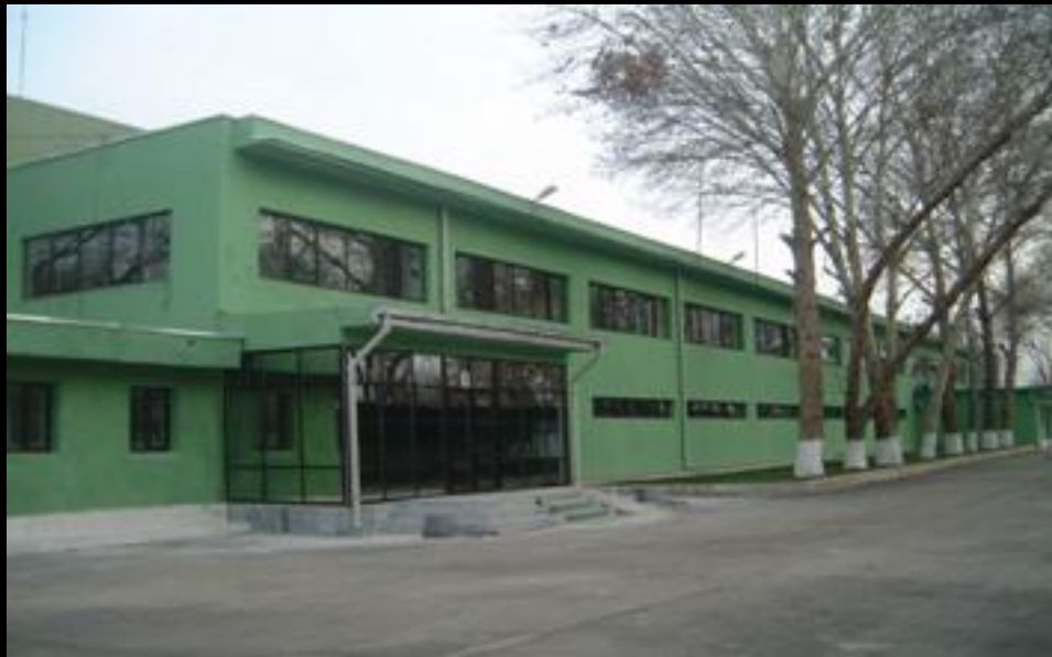
Project Name: Demir Textile Yarn and Weaving Factory Year: 2004 Scope of Business: Key Contract Size: 15,000 sqm Location: Tashkent/ Uzbekistan
