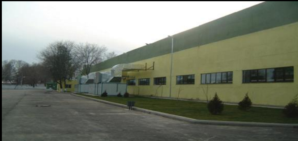
Project Name: Yadem Textile Knitting, Dyeing, Apparel Factory Year: 2002 Scope of Business: Key Contract Size: 17,500 sqm Location: Tashkent/ Uzbekistan
